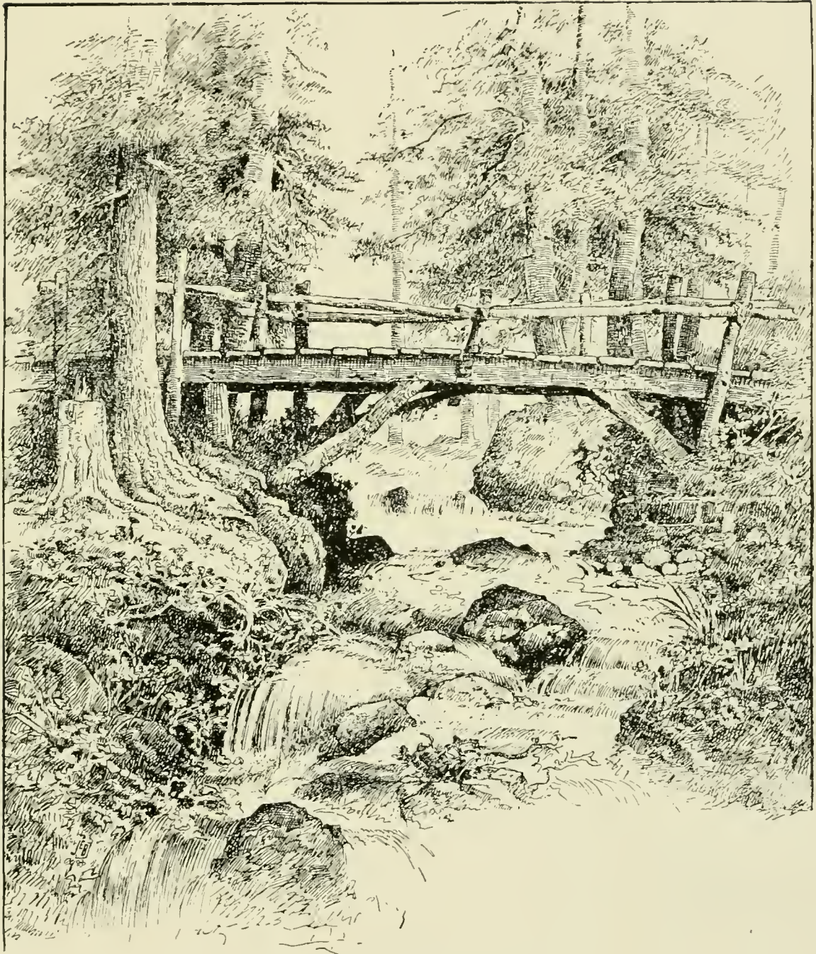
THE STAID WOODEN BRIDGE.
